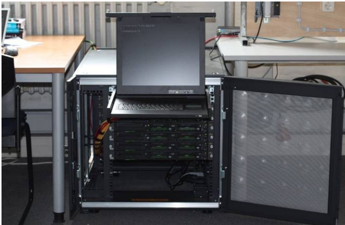
Smart Grid Control Center
