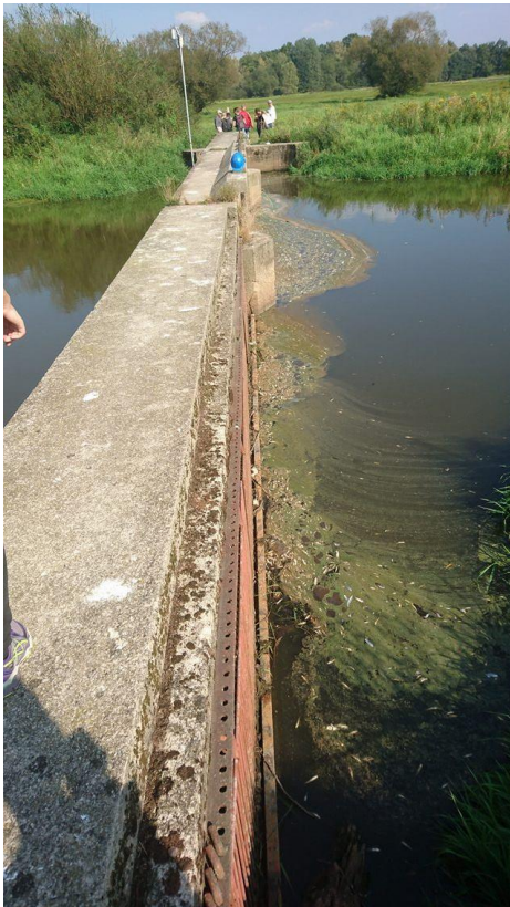
Fig 2: Artificial channel for water regulation in wet meadows and fishponds (photo by Mari Oll)
