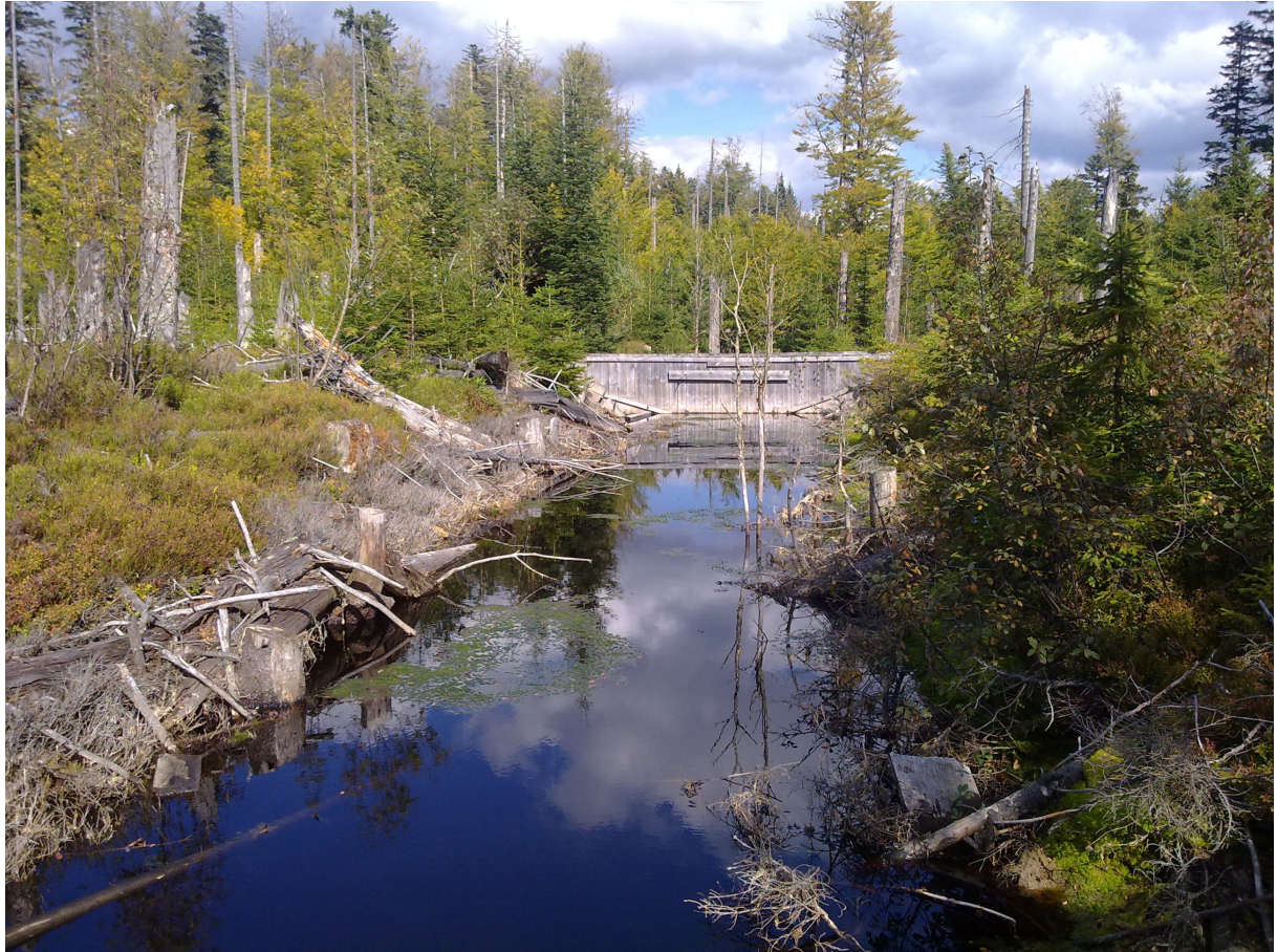
Figure 5: Large ditches in peat bogs with dams to prevent water flow and drainage
