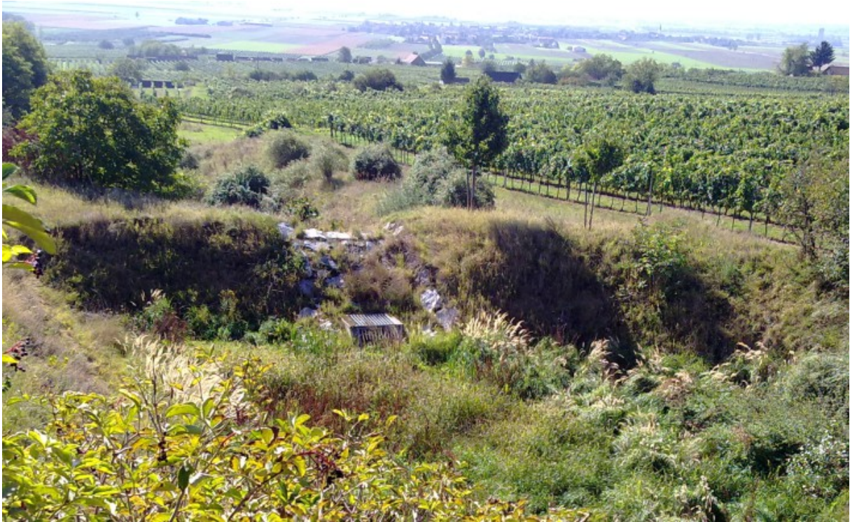
Figure 3: Construction works between vineyards for erosion prevention
