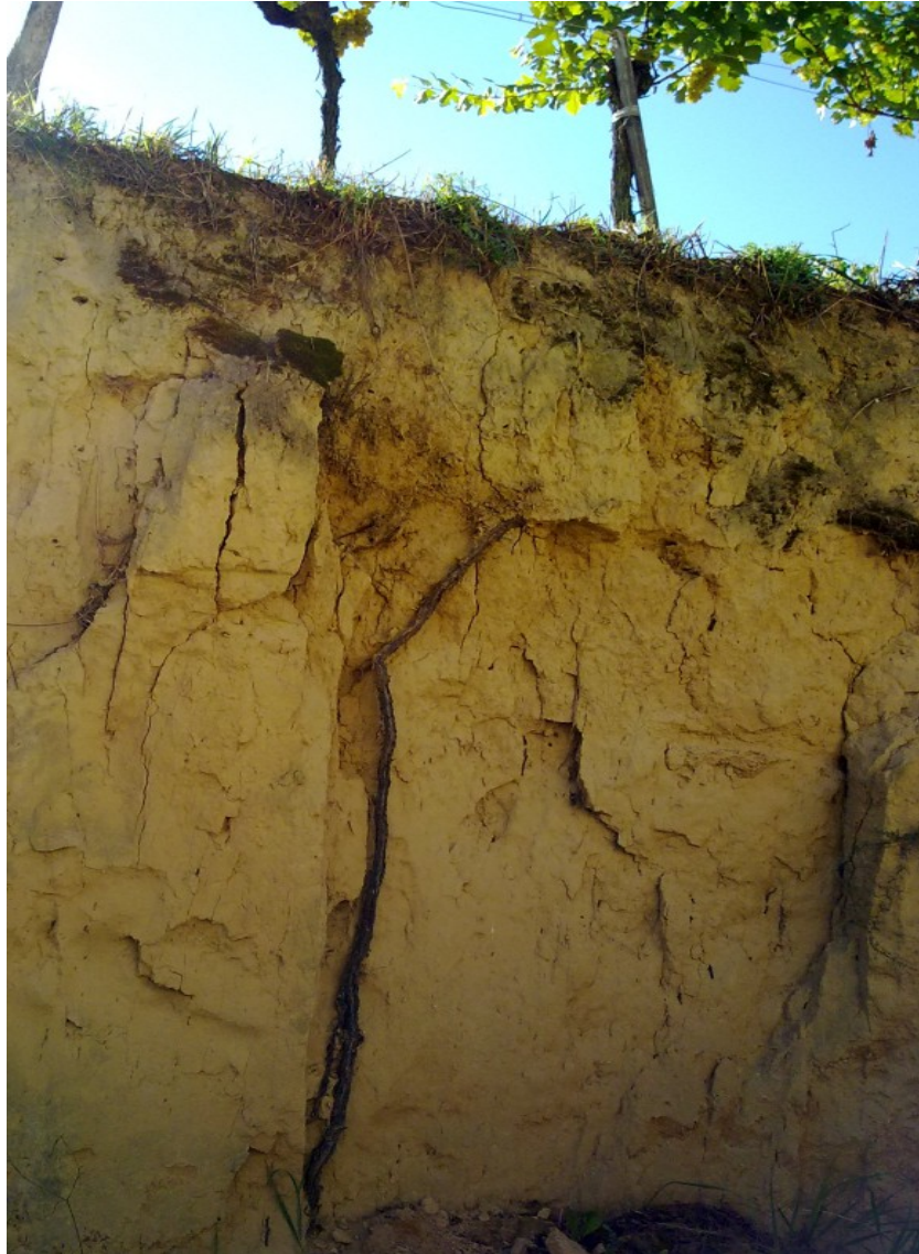
Figure 2: Deep roots are visible on edges and in hollows created by erosion
